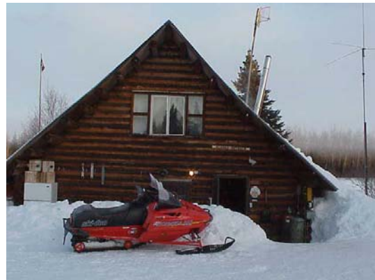
Checkpoint Building: Skwentna
